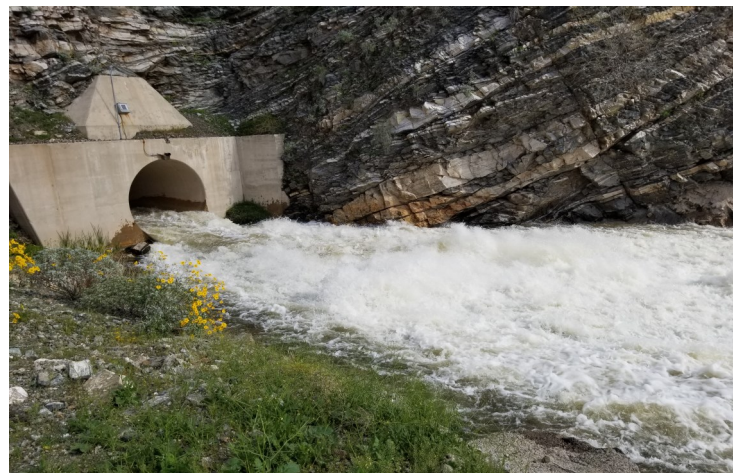
Alamo Dam Outlet Works. The flow shown here is about 500cfs above the normal base flow amounts. Photo Courtesy of Jim Boyd
